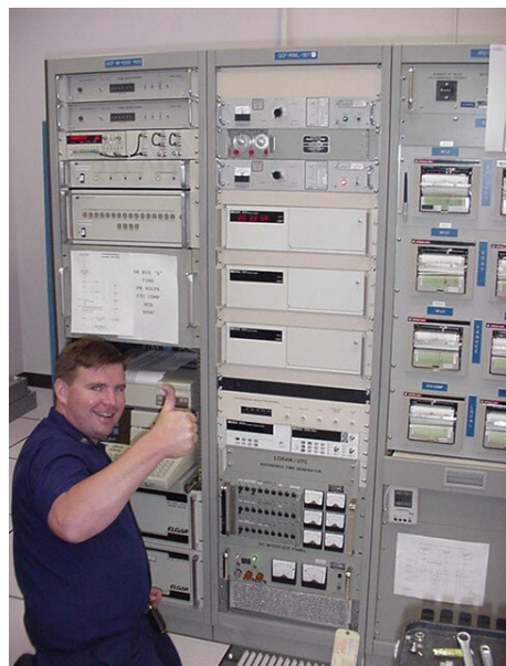
Figure 7: New Cesium Beam Oscillators and TTM Equipment (LORSTA Havre, MT)
