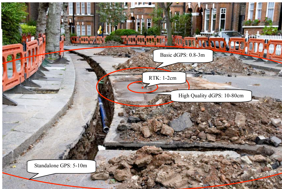
Figure 2: Attainable accuracy by receiver type from an OS Net based partner correction source.
