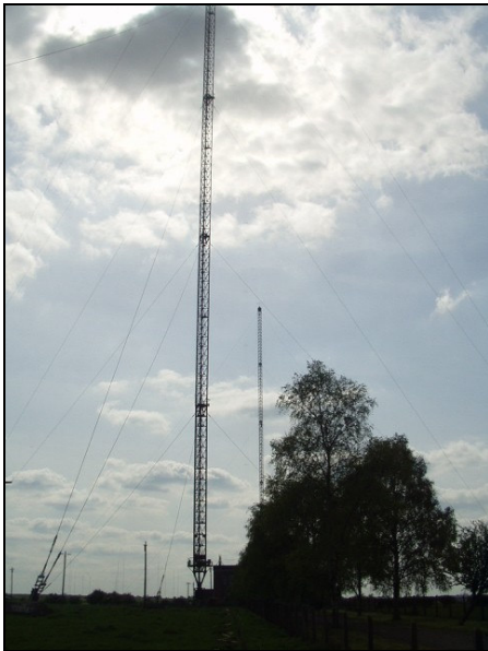
Fig. 2 – The two masts used to support the Loran antenna.
